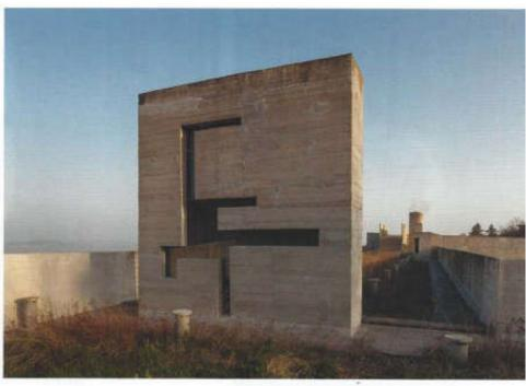
Above left: lannis Xenakis, a musician and Le Corbusier's assistant, designed the undulating glass surfaces. Above right to light this stairwell, a design resembling the blade of a key was cut into the reinforced concrete
